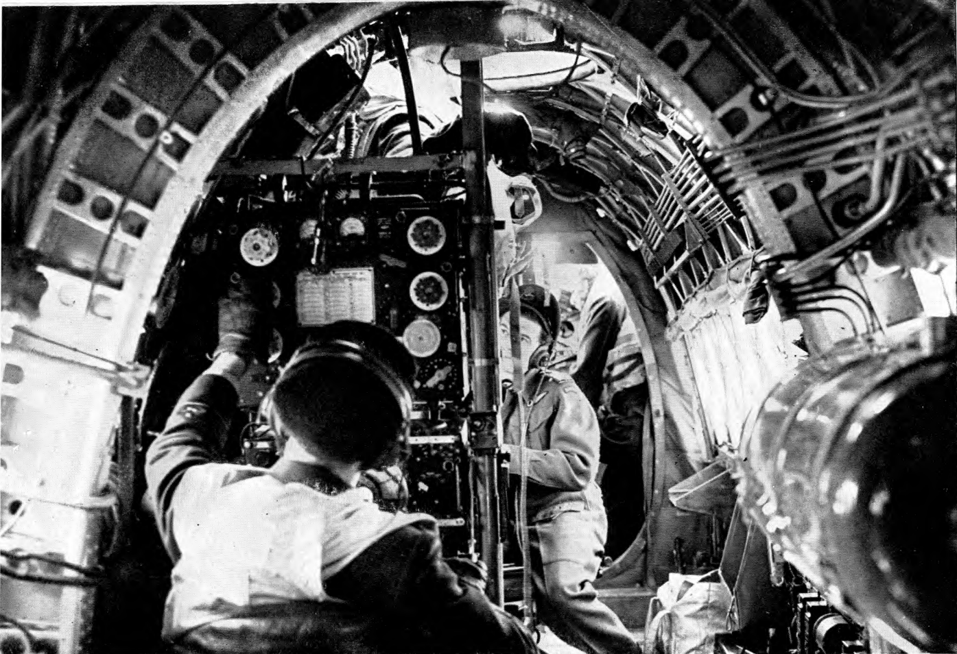
Interior of the Warwick transport, showing the flight engineer's panel.
