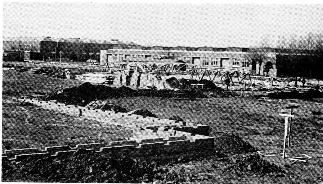
5(T) Block being built, 1967. The Station Gym is in the background.
