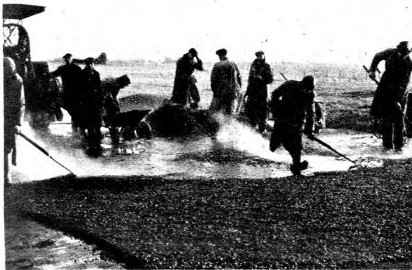
Construction: British labor works on a field for Forts.
